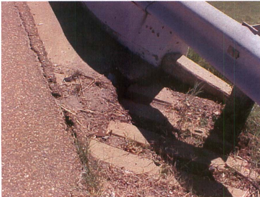
APPROACH #1, RIGHT DRAIN IS BROKEN
