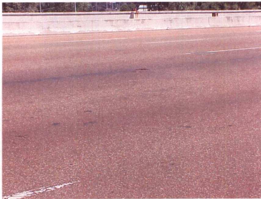
SPAN #1 WITH ASPHALT SPALLING
