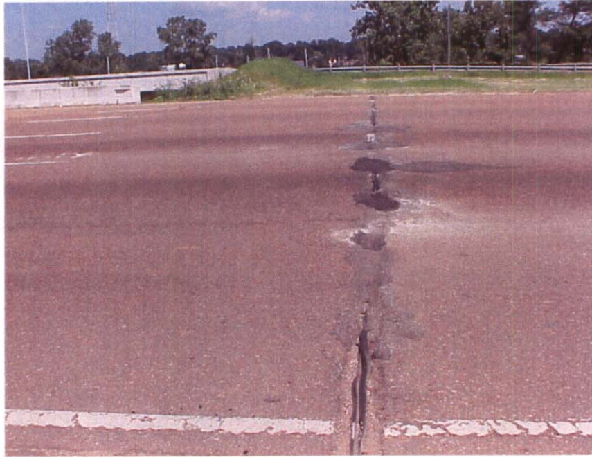
APPROACH #2 JOINT HAS UNEVEN ASPHALT
