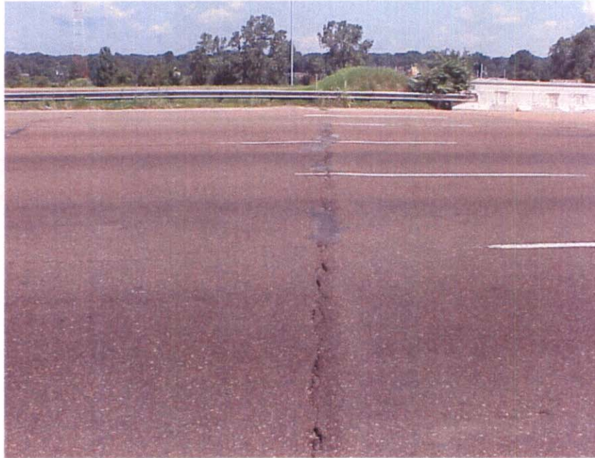
APPROACH #1 JOINT HAS ASPHALT CRACKING & SPALLING
