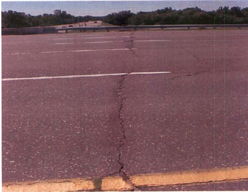
APPROACH #1 PAVEMENT SPALLING
