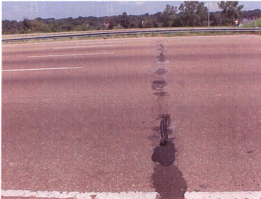
APPROACH #1 JOINT HAS ASPHALT CRACKING & SPALLING
