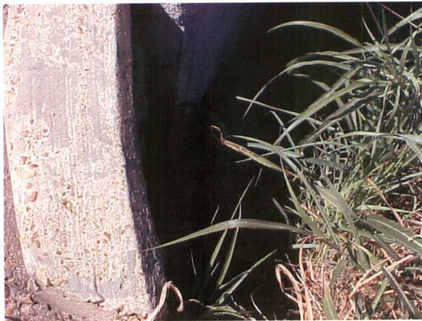
APPROACH #2, LEFT EMBANKMENT WASHING
