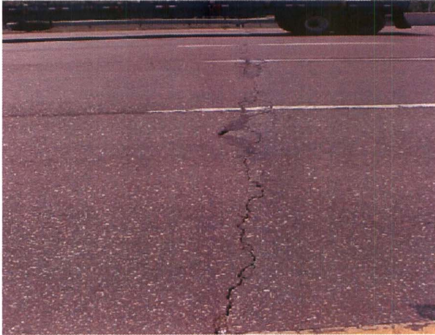
APPROACH #2 PAVEMENT CRACKING & SPALLING
