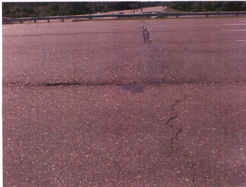
APPROACH #1 JOINT MATERIAL MISSING
